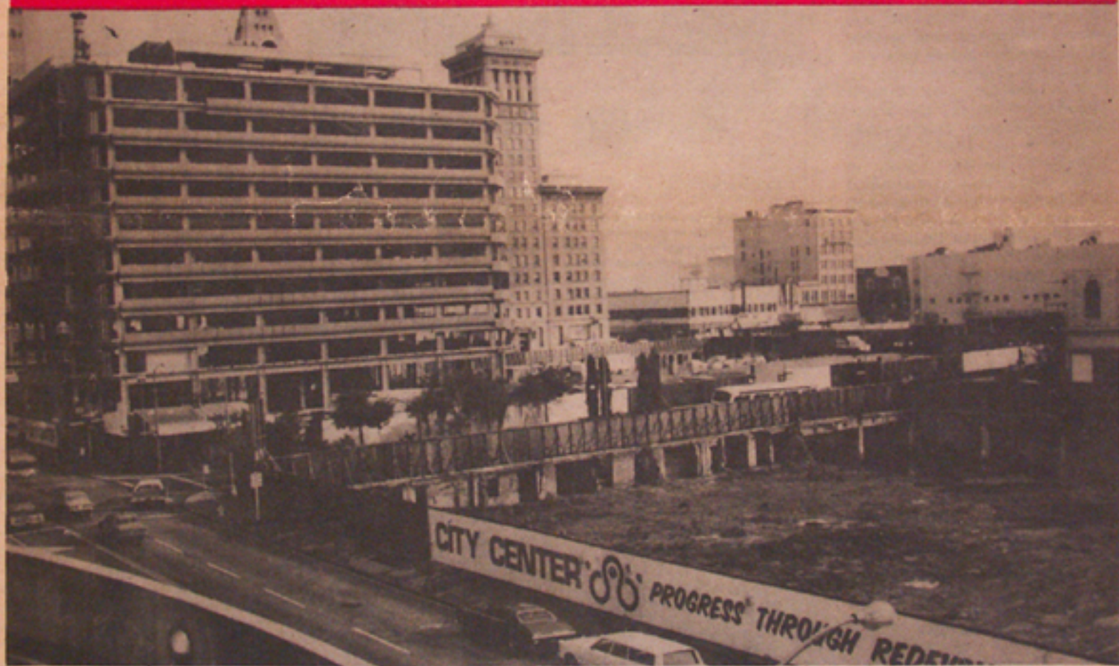
City Center Project construction sites.
